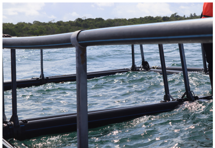
IMTA Cage under construction in Kijiweni, Kwale County.
